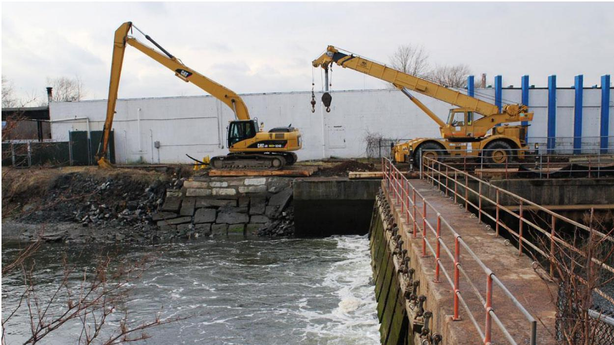
**Figure 1-2.** Tide gates at New Haven partially separate the West River (shown here) and the Mill River from Long Island Sound. CT Fund for the Environment/Save the Sound and partners have modified the gates to partially restore tidal flow. ([newenglandboating.com](http://newenglandboating.com))
