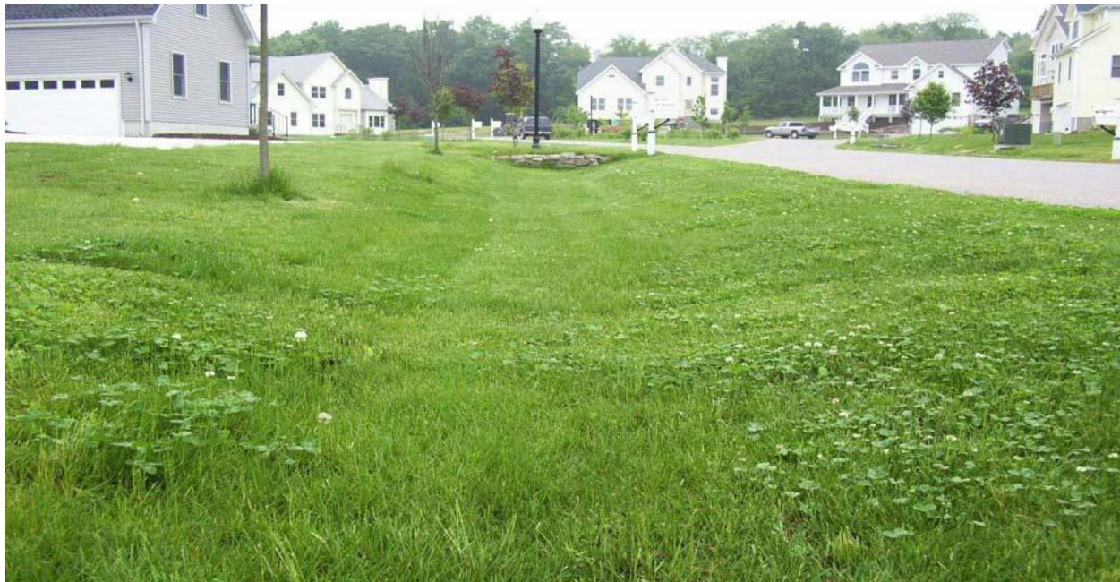
**Figure 3-9.** Low impact development (LID) on a dry day. This neighborhood does not need storm drains and rain filters through the soil to recharge local water supplies. (University of Connecticut)
