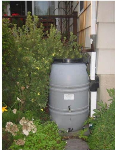
Rain barrels collect water from a roof downspout and hold it for later use.
