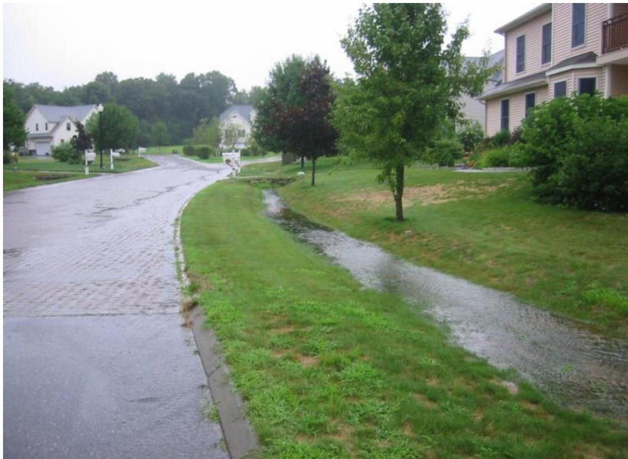
**Figure 3-8.** A low-impact development (LID) uses landscape features like grassy swales instead of storm drains to collect and filter water on a rainy day. This design greatly reduces water pollution and recharges underground water supplies. (*University of Connecticut*)
